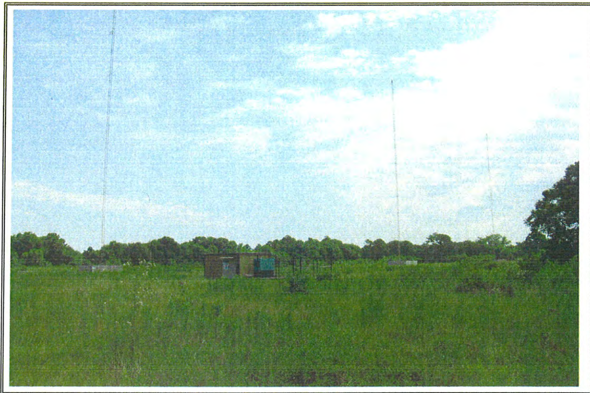
Photograph Number 2: View depicts communication towers observed at the project site.
