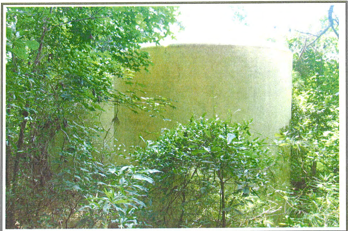
Photograph Number 4: View depicts example plastic AST observed at the project site.
